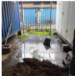
The Dalton mess begins to seep in
